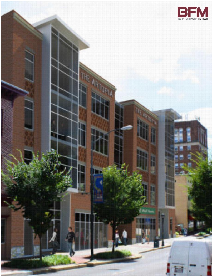
Buildings 1 & 2—Potomac St. Façade
