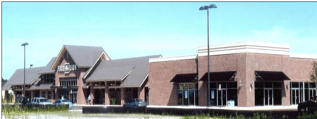
Sample of architectural articulation required of Destination Retail Use Buildings. The larger store on the left has architectural articulation as described. Compare this storefront with the smaller store on the right which is not articulated and appears proportionately larger.
